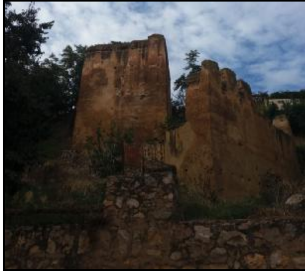
Figure 36: Bordj Essoltane, Source: l'auteur
