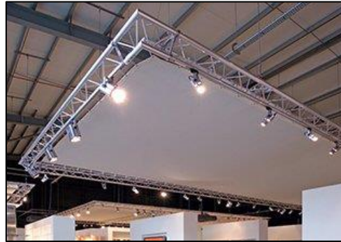
Figure 138: un stand en structure aluminium.
