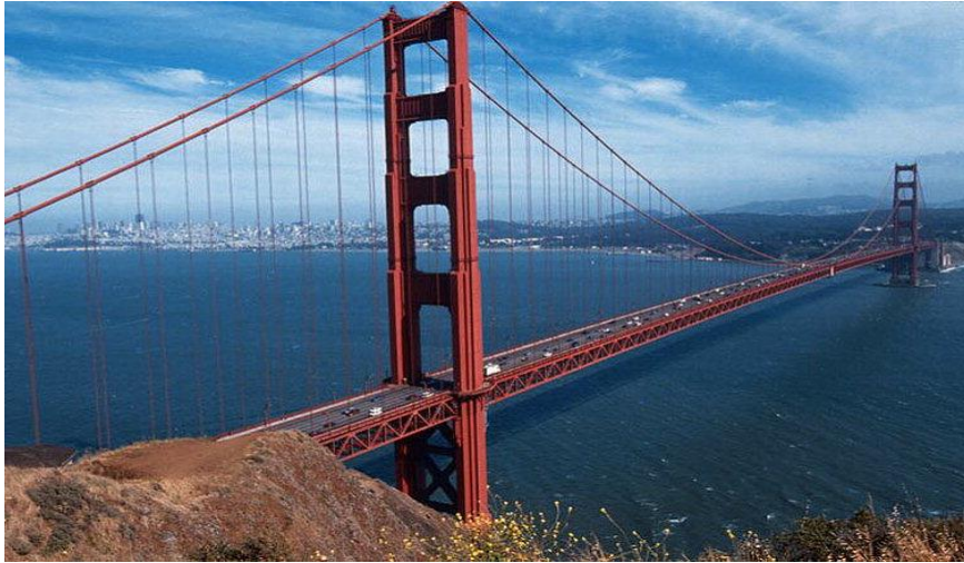
Figure I-6 : Golden Gate bridge
