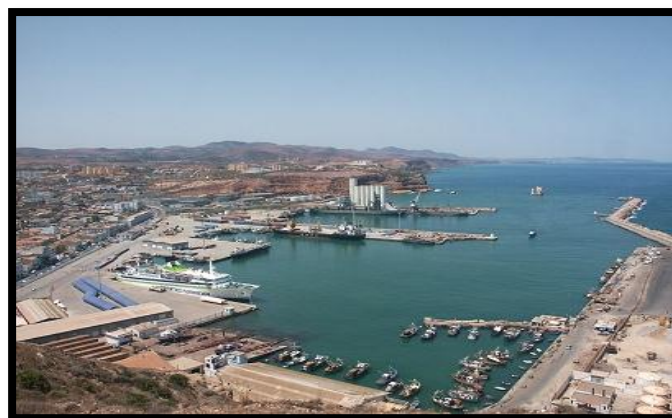
Figure 64: port de ghazaouete
