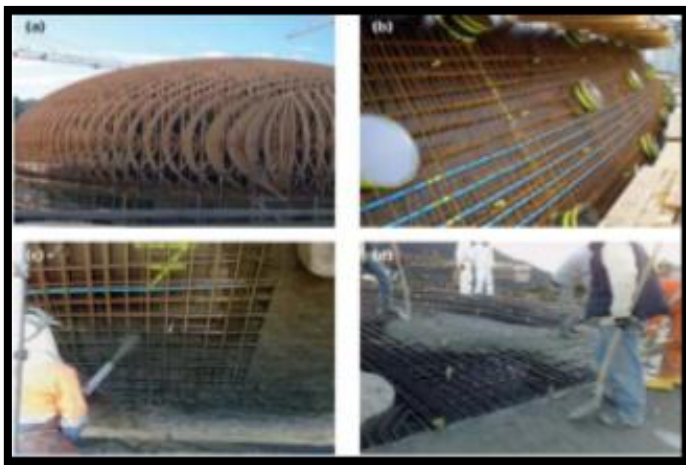
Figure 95: construction de la coque
