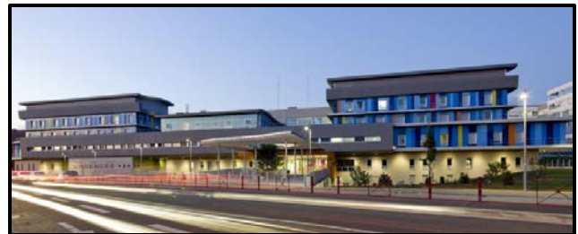
Figure 22 : la façade principale
