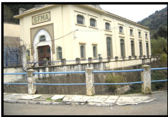
Figure 010: La centrale hydraulique de Boghni Source: http://www.dircultureto.dz
