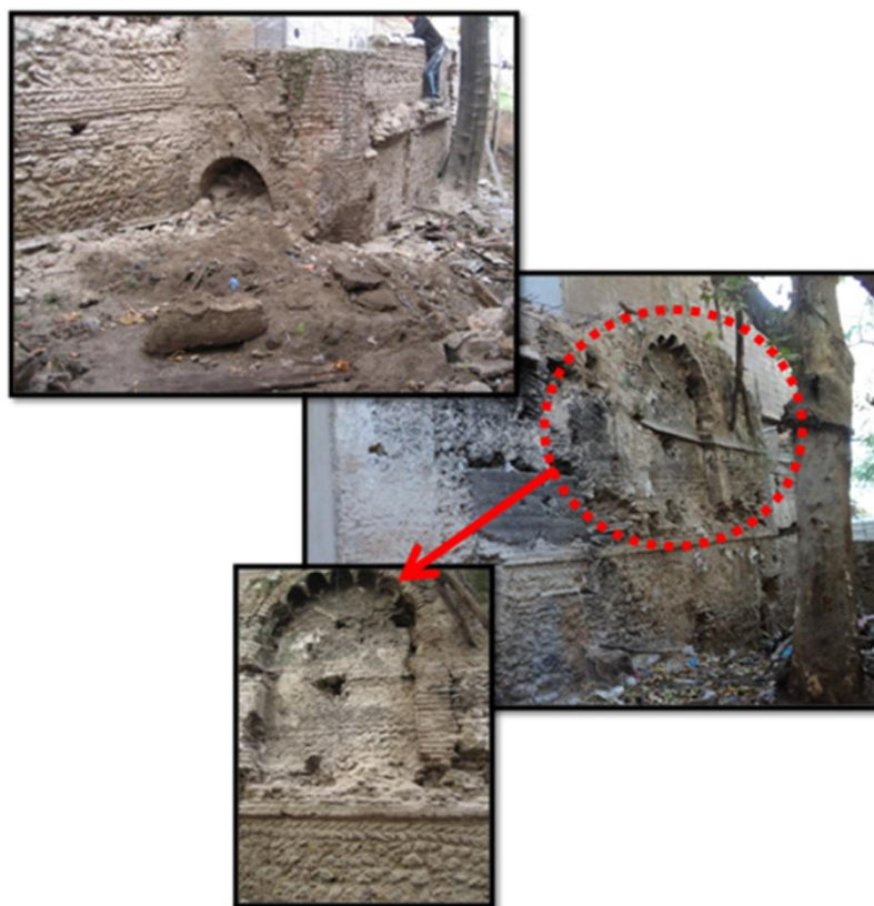
Fig.45: Murs de Bab El Quaysaria Source: OGEBC
