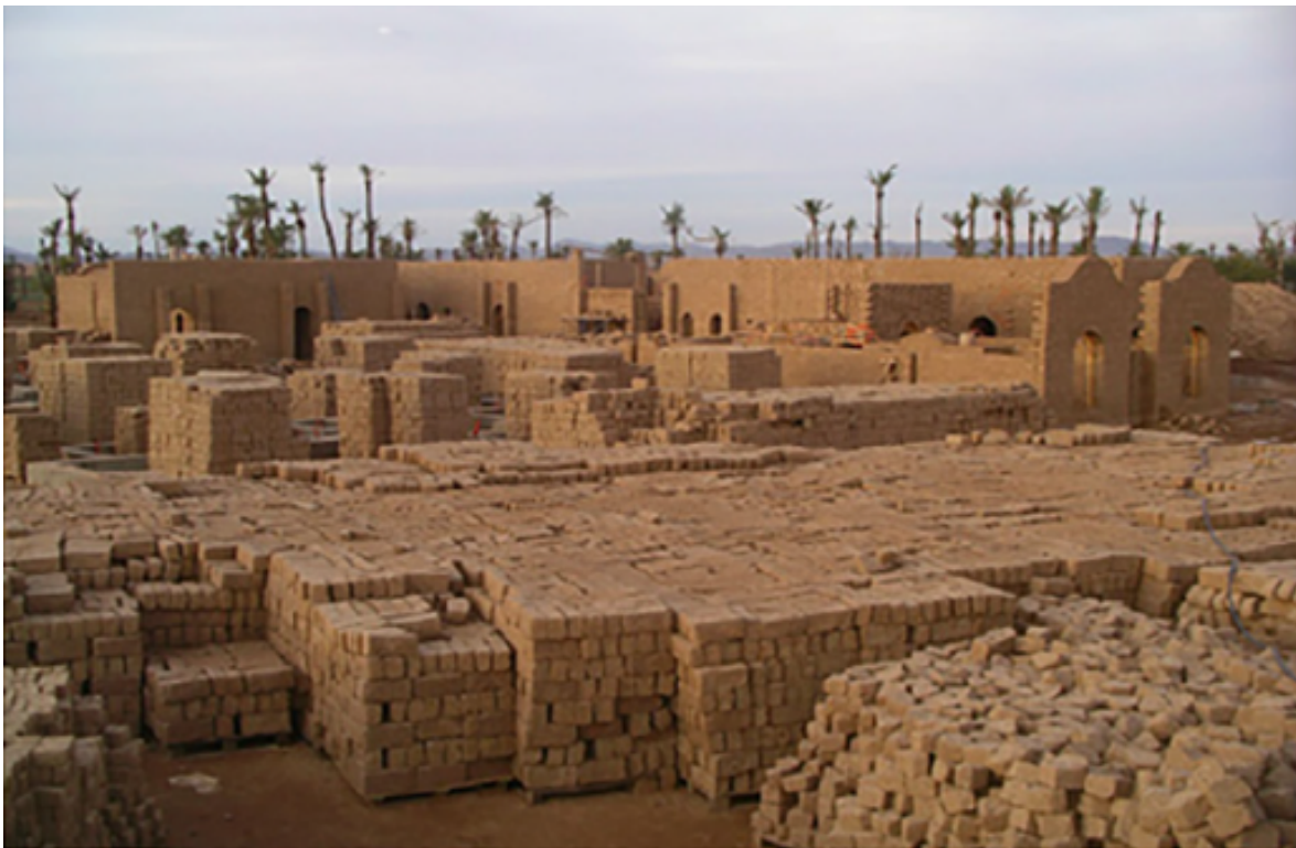
FIGURE 4.11 – Stockage massif d'adobes, Villa Janna, Marrakech, Maroc, [Van-Damme and Houben, 2017].
