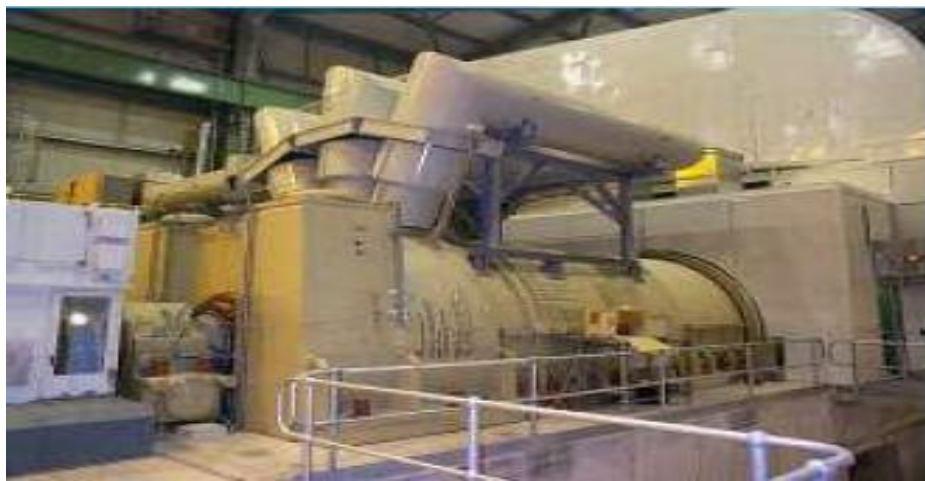
Figure (II. 20) Alternateur 50WT21H-120
