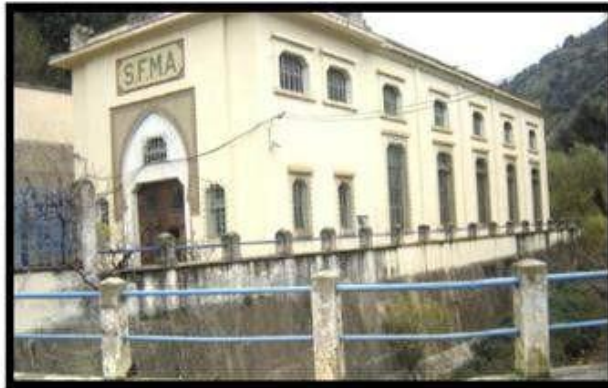
Figure 8: La centrale hydrolique de Boghni (tizi-ouzou)
