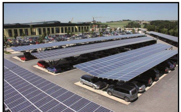
figure 173: parking solaire photovoltaïque
