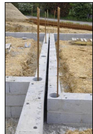
Figure 119: joint de rupture
