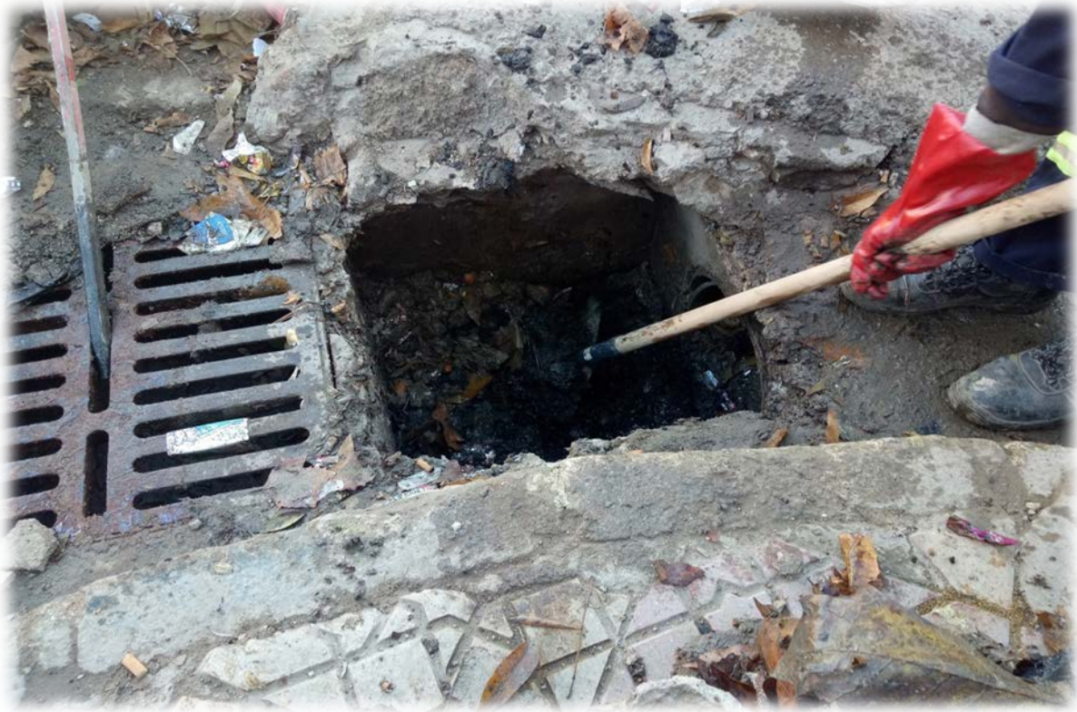
Figure III.5 : Curage manuelle.
