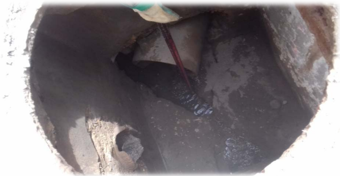
Figure III.35 : Branchement irrégulier.
