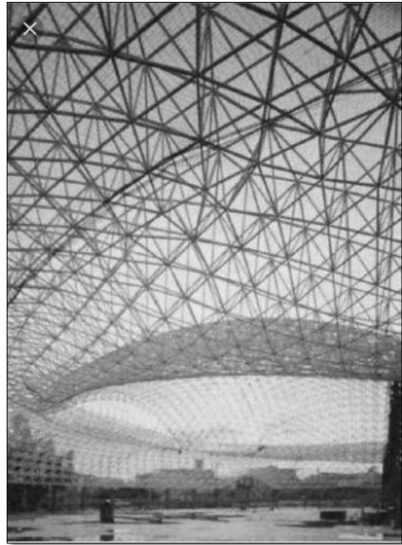
Figure 55: gridshell de Palafolls Sports Hall
