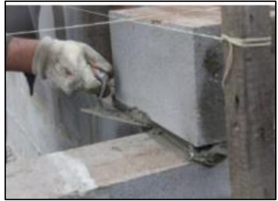
Figure 146: Cloisons en parpaings
