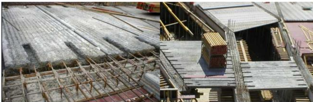
Figure II.1 : Plancher corps creux
