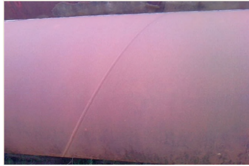
Figure I.34: soudure spirale (STT)
