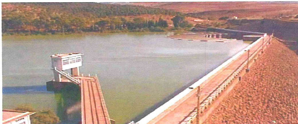
Figure 16 : Barrage Dahmouni (original ., 2017)
