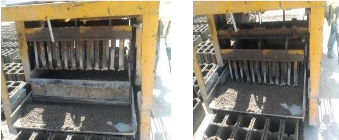
Figure III.6: compactage par vibration.
