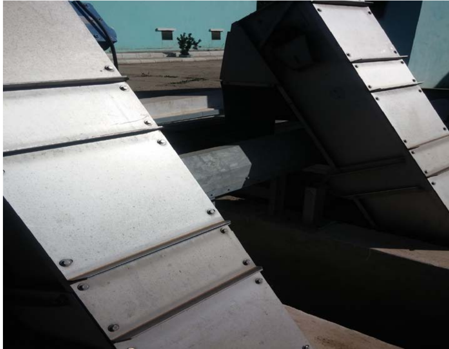
Figure III. 2: photo des grilles grossières
