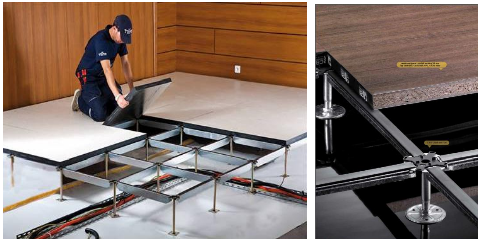
Figure 88: les planchers Techniques
