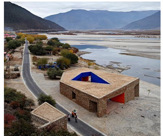
FIGURE28 : niyang River Visitor Center
