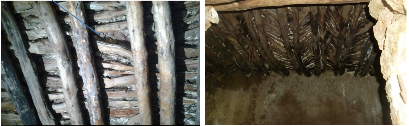
FIGURE 78: solives supportant le plancher
