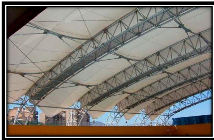
Figure 78:structure tendu câble membrane a arc
