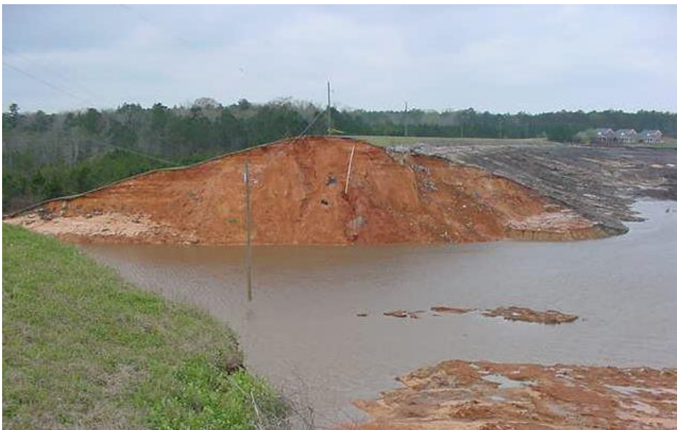
Figure 3.19: Rupture de barrage de Big Bay (Internet)
