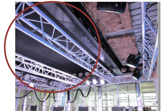
Figure 4: photo montrant la passerelle
