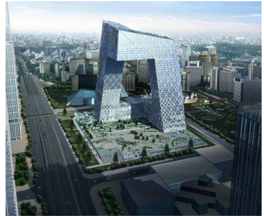
Figure 22 Centre de CCTV
