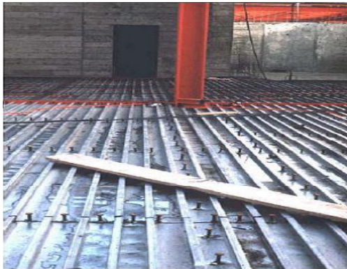
Figure: plancher collaborant
