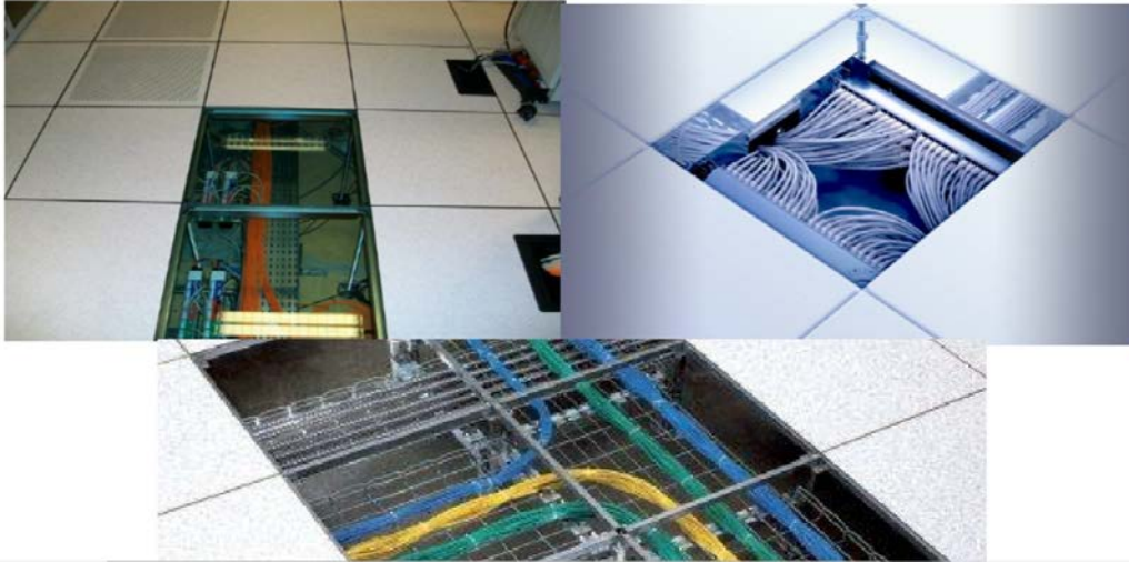
Figure 150: les planchers techniques
