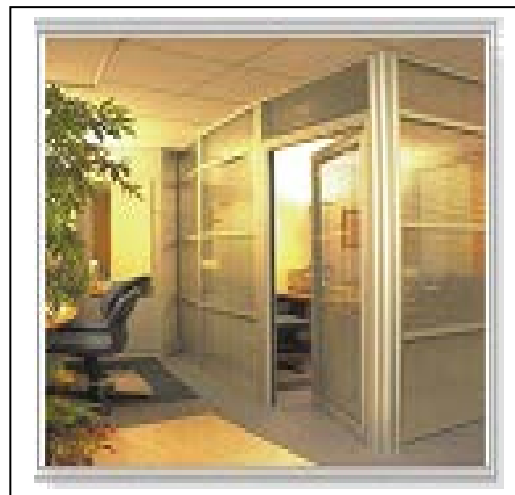
Photo 23: cloison vitrée
