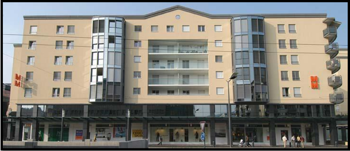
Figure 68: Façade principale midi coindet source : wéb 59
