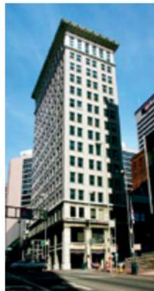
Figure 14:immeuble Cincinnati, USA, 1903
