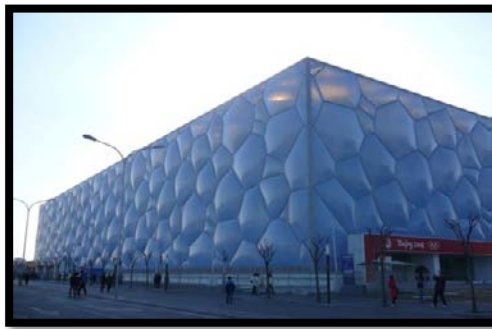
Figure n 17: structure gonflable
