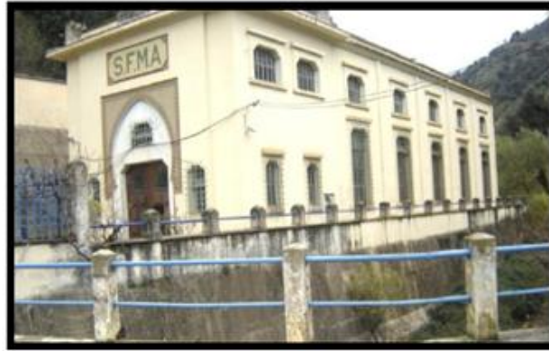
Figure 8: La centrale hydroliqye de Boghni (tizi-ouzou)
