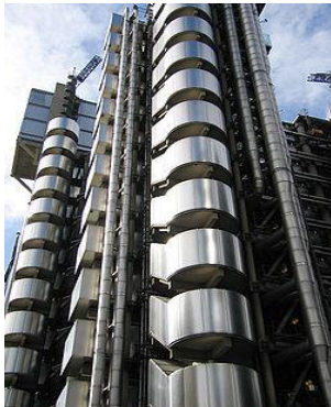
Figure 19. Le Lloyd's Building, Richard Rogers
