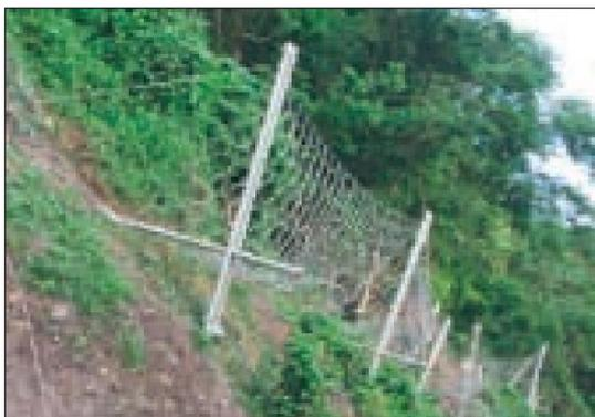
**Figure 182.** Filets pare-blocs.
