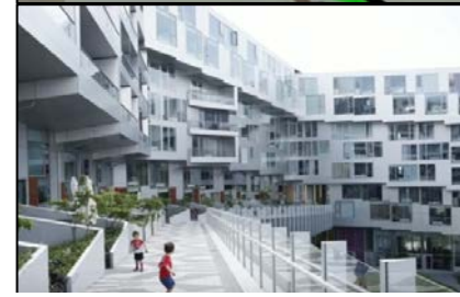
Figure 44 the 8 house. Source : archdaily
