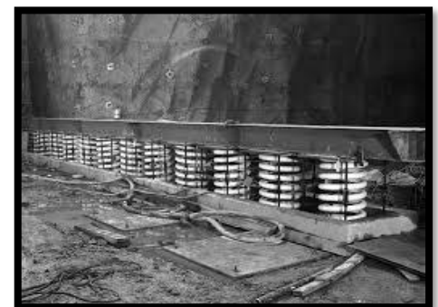
Photo 47 : Ressort anti sismique http://www.abovetopsecret.com/forum/
